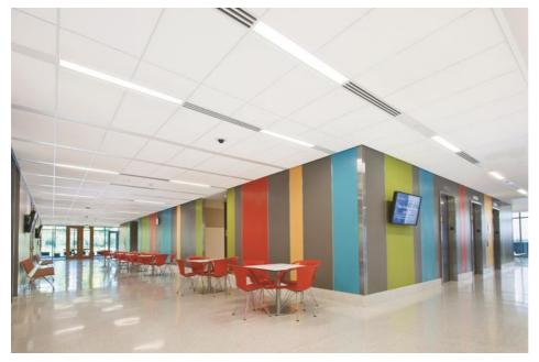
Inconspicuous integration of technical components: The TROX slot diffusers made of high-quality extruded aluminium sections blend in perfectly with the TECHZONE  $^{\rm m}$  ceiling system.
