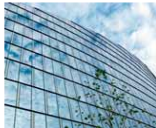
Main-Triangel, Frankfurt/Main Architect: Architect Group N+M GmbH, Offenbach Specialist consultant: Pettersson + Ahrens Construction company: Kretz + Wahl Gebäudetechnik GmbH & Co. KG
