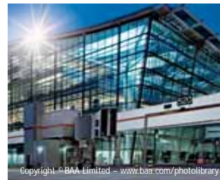
Terminal 5, London Heathrow Airport Architect: Richard Rogers, Rogers Stirk Harbour + Partners, London Specialist consultant: WSP Consulting Engineers Construction company: Amec Building & Facility Services – MACE
