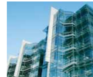
Chambre de Commerce, Luxembourg Architect: Claude Vasconi & Partners, Paris Specialist consultant: RMC Consulting Construction company: ELCO S.A. – ABB Luxembourg – Climalux S.A.
