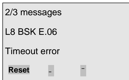
Figure 6.12.2: Fire damper message with a customer-specific designation in line 2
