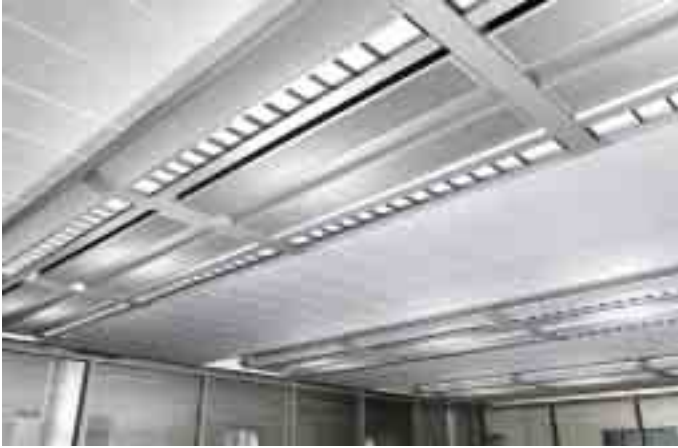
illustration 16 – glass partition intersecting MSCB.
