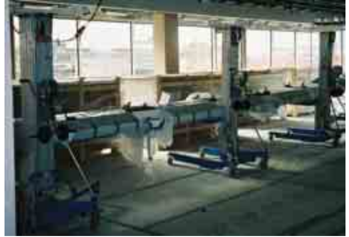
illustration 13 – MSCB positioned on 'Genie' hoist prior to fixing.
