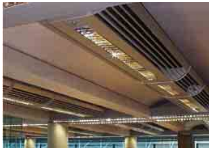
illustration 25 – section through exposed passive MSCB at Lloyd's Register of Shipping.
