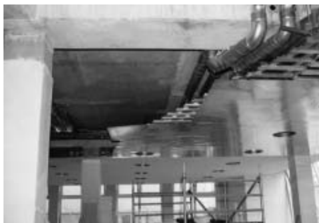
Figure 5: Chilled ceiling for plastering
