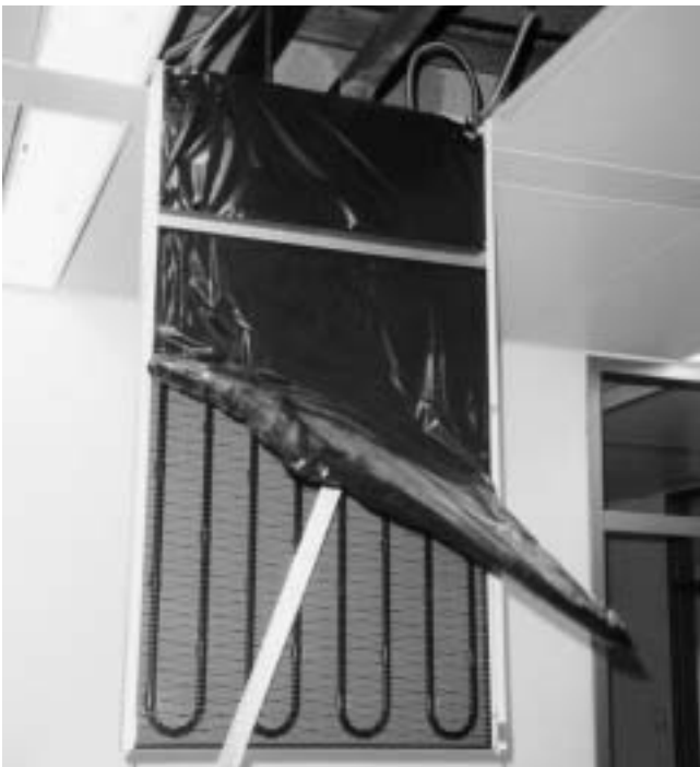
Figure 2: Pivotal chilled ceiling element WK-D-UM (e.g. for inspection)
